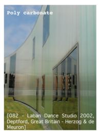
The polycarbonate plates come in different colors and be easy to find in the area. They give an interesting facade with different colors. It is a light material both in weight and expression and is isolating noise.
