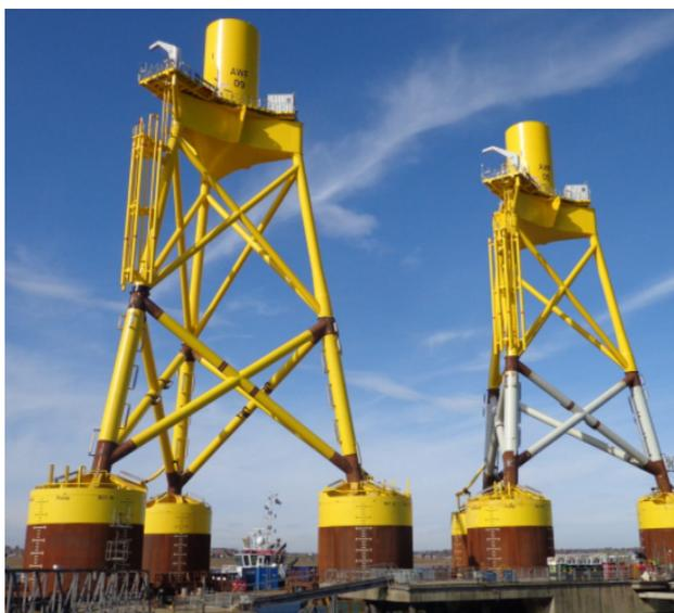
**Figure 1.2:** Suction bucket for jacket structures- (SPTOffshore, 2021)
