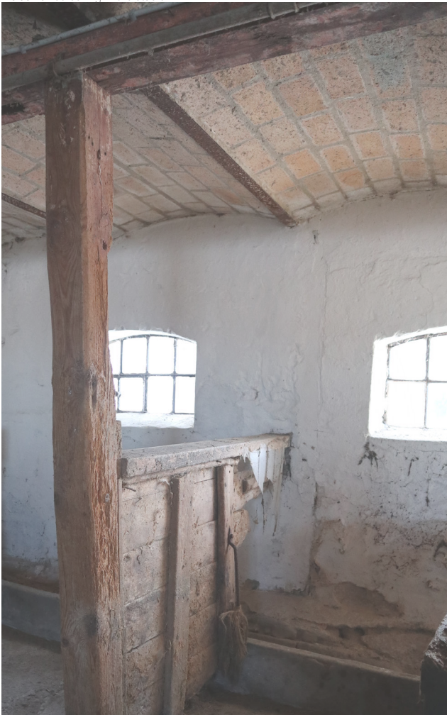
FIG.08 Valved ceiling in the stable
