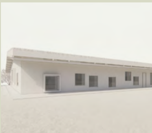
Facade option 5 - Fits to the grid system and provides an average daylight factor above 2.5%
