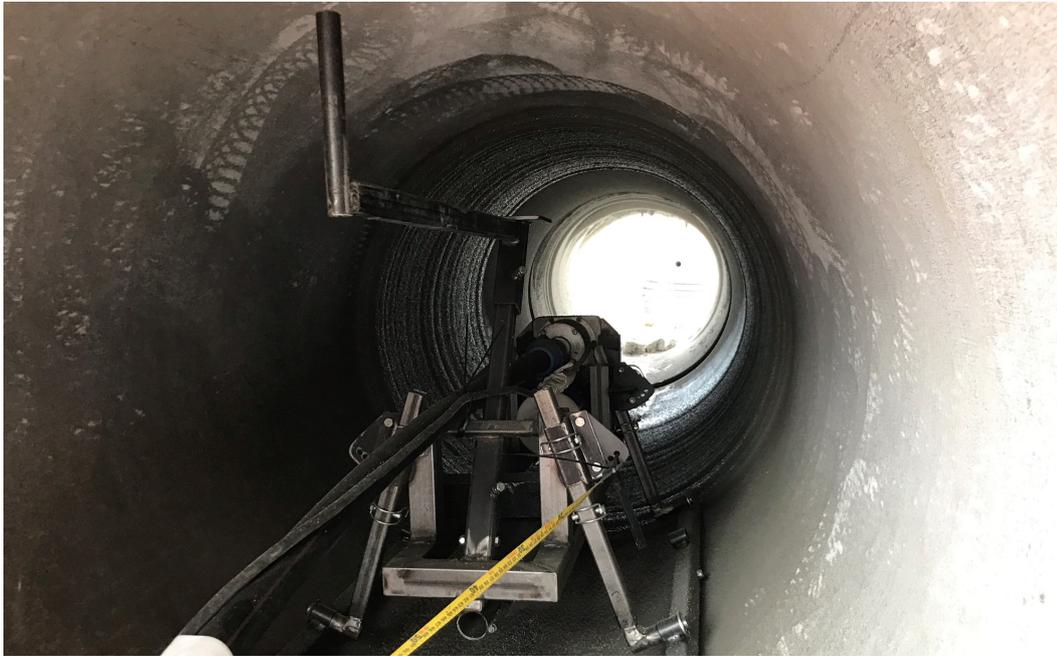
**Figure 1.1:** Concrete spraying machine at a test site with freshly sprayed concrete.
