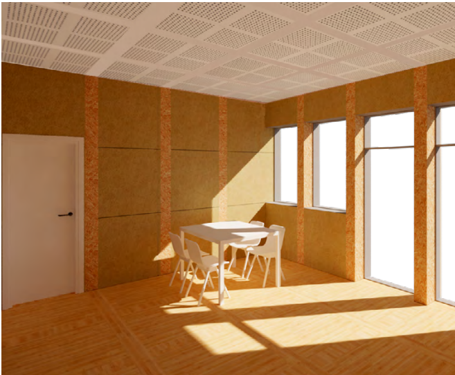
Illu 218: Clay, particle board, bamboo and gypsum Daylight factor: 2,8% Reverberation time average 125-4000Hz: 0,4s
