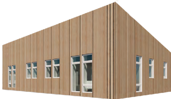
Illu 272: Natural ventilation 5. Mullions separating the tall windows
