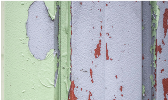
054. Photo Gables of the block clad with painted zink in a renovation
