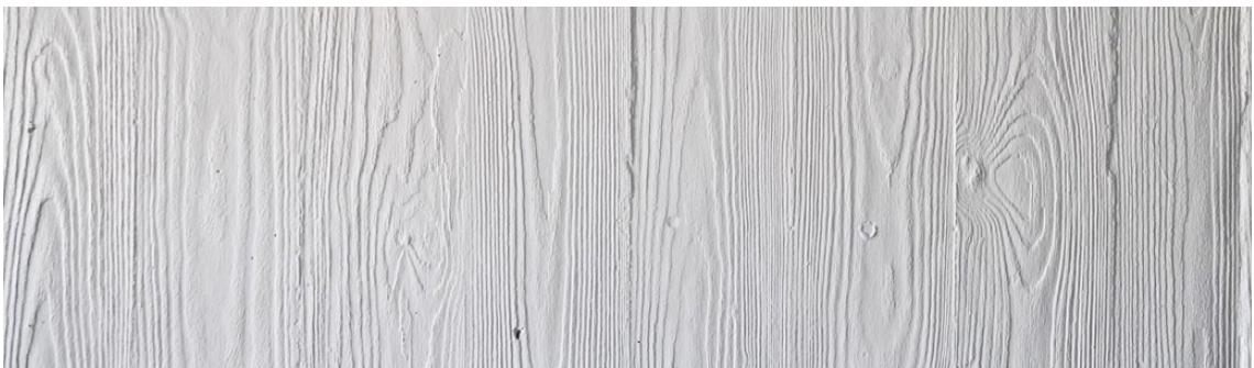
051. Photo Concrete with cast of its wooden formwork
