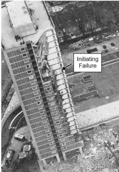
**Figure 2.1:** Progressive collapse of the corner of Ronan Point.
