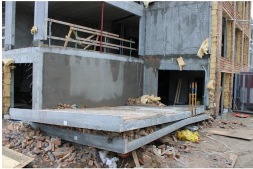
**Figure 5.1:** Image from the Da Vinci failure. Image: Nordjyske Stiftstidende [2019].
