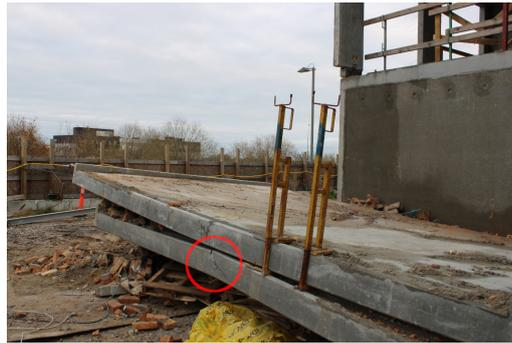
**Figure 5.2:** The Da Vinci collapse with the crack in the slab circled in red. Image: Nordjyske Stiftstidende [2019].
