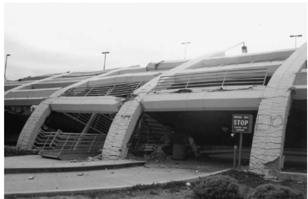
Figure 1.2: Parking structure that collapsed during the 1994 Northridge earthquake, California State University, Northridge Campus[Erdey, 2007]
