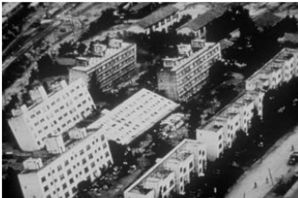
Figure 1.1: Damage to apartment buildings caused by soil liquefaction during the June 16, 1964, Niigata (Japan) earthquake[Seth Stein, 2005]
