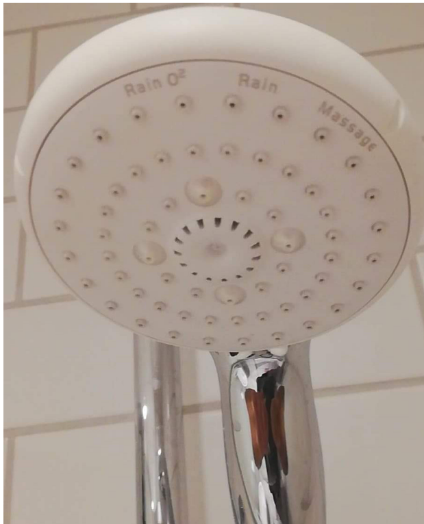
Picture 28. Showing three dif- ferent low pressure modes (Rain O2, Rain and Massage)
