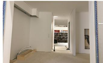
3 Figure 5.4: Interior gypsum plates and paint
