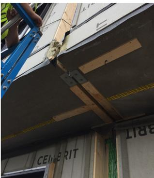
Figure 5.14: Vertical connection
