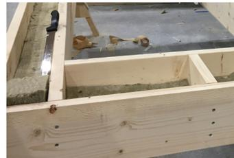
6 Figure 5.7: Insulation on the wall
