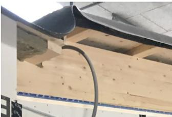
4 Figure 5.5: First layer of roof
