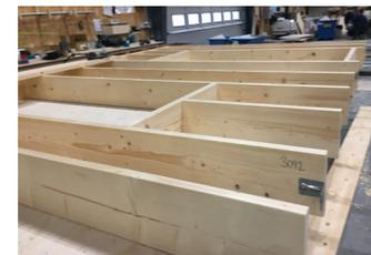
7 Figure 5.8: Second layer of exterior wall
