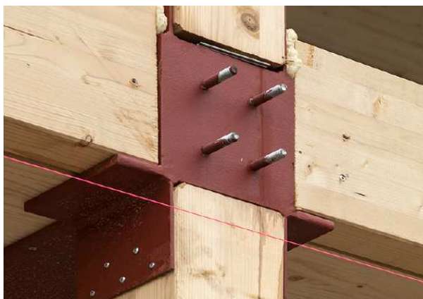
Ill. 27 Joint. Column and beam connection in Lisbjerg Bakke
