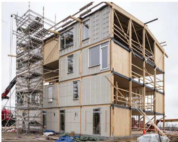
Ill. 26 Wood cassette fixed to the skeleton construction
