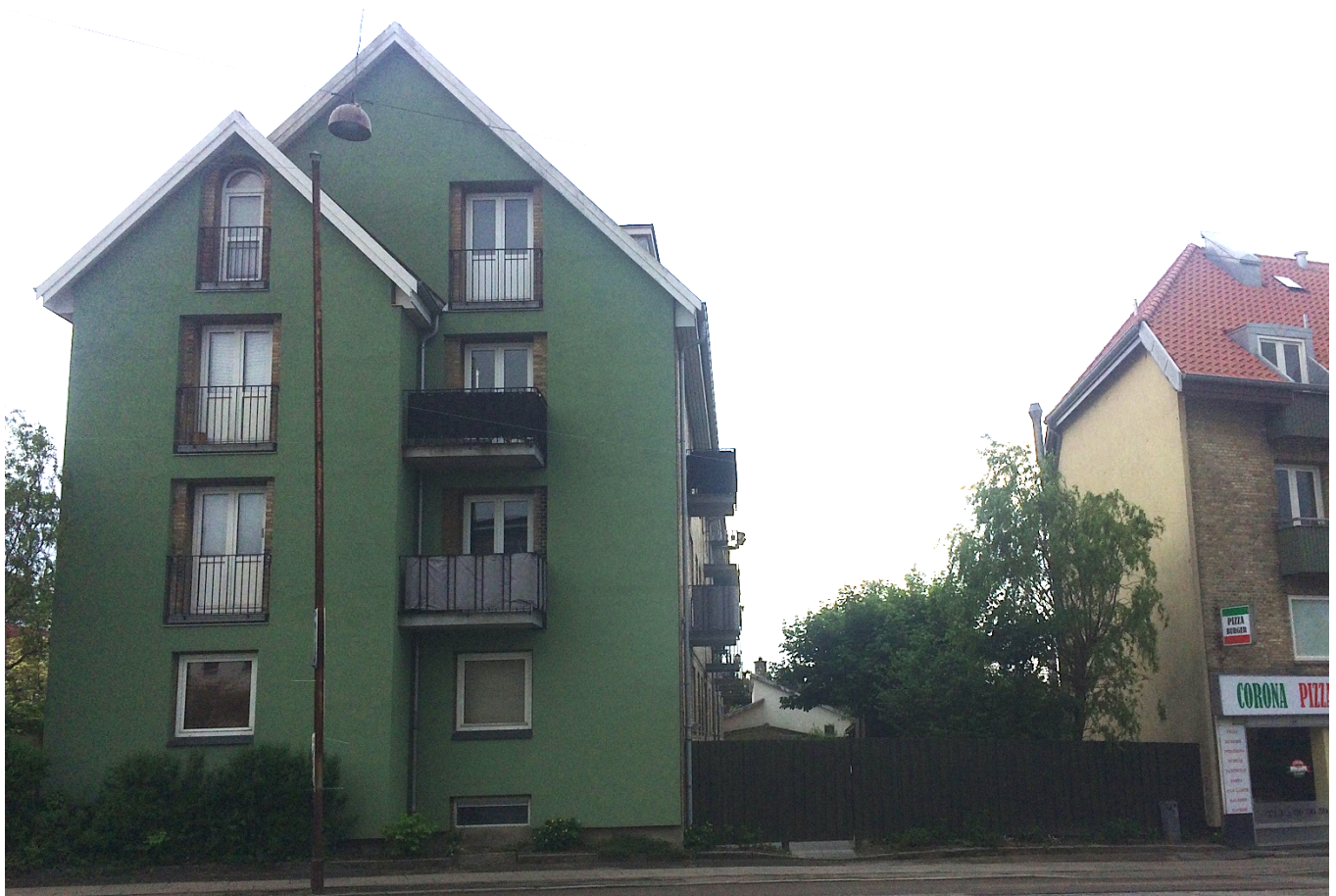
Figure 1.7: Two examples of façade renovation in Søborg, Copenhagen. The left building looks clumsy and does not remove all line-losses, since insulations and render does not reach the doors. By author
