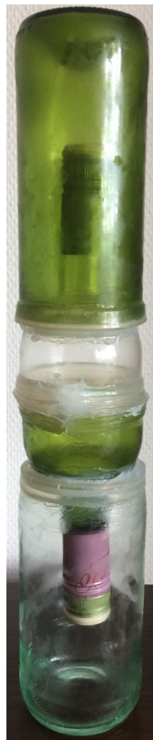
Figure 2: Three air compartments separated with rubber seal and silicone arguably makes this wine bottle-brick insulated.
