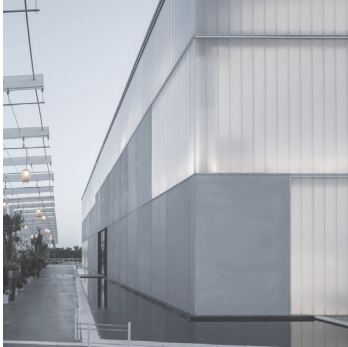
III. 103 - Double-glazed facade solution
