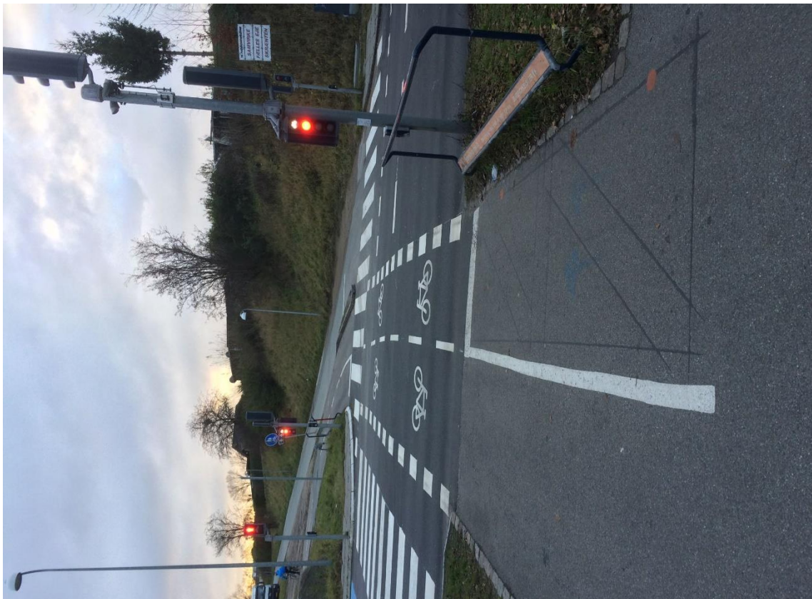
The crossing with Klausdalsbrovej. The sensors can clearly be seen. By riding over the sensors, the cyclists get a green light and can carry on cycling without stopping. This is not an ideal location to hand out survey invitations. Source: Arne Kempers, 2018.
