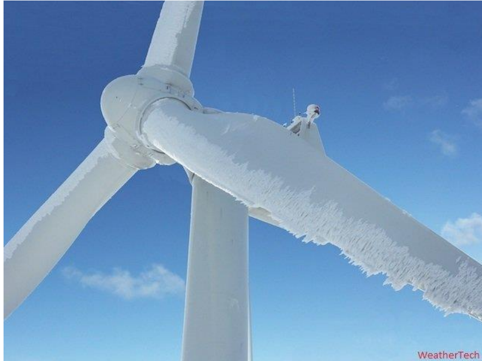
Figure 2. Icing effects on wind turbine [4]
