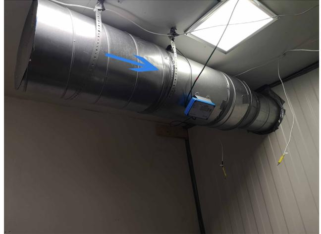
**Figure 5.6:** Lindab Ultralink supply airflow direction - cold room
