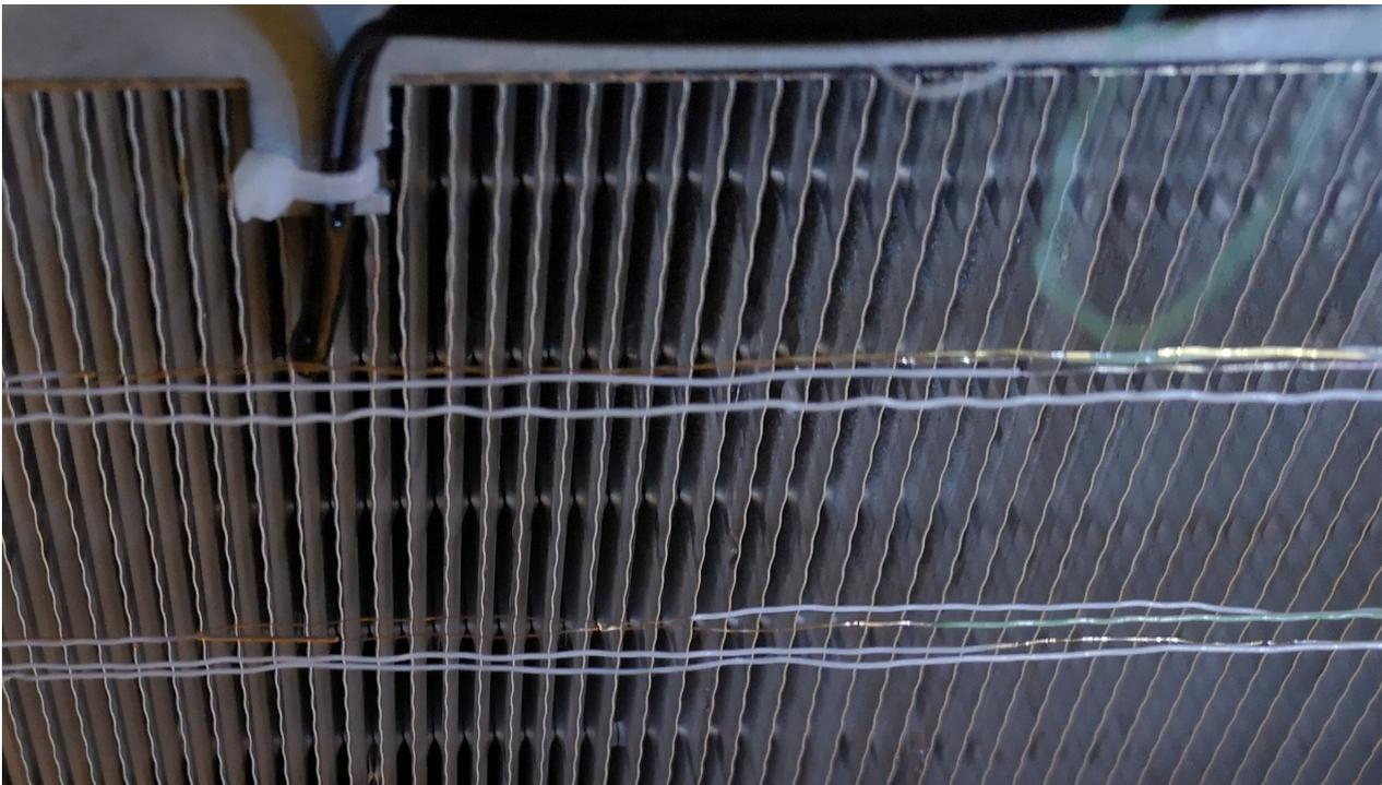
**Figure E.7:** Small droplets of condensation at second 1000 - condition 2
