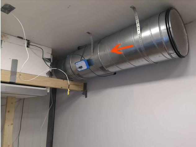
**Figure 5.5:** Lindab Ultralink extraction airflow direction - warm room
