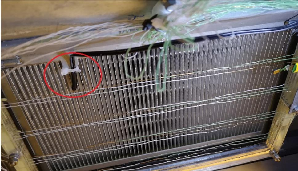
**Figure 7.9:** Airmaster's temperature sensor on exhaust port (marked with a red circle)
