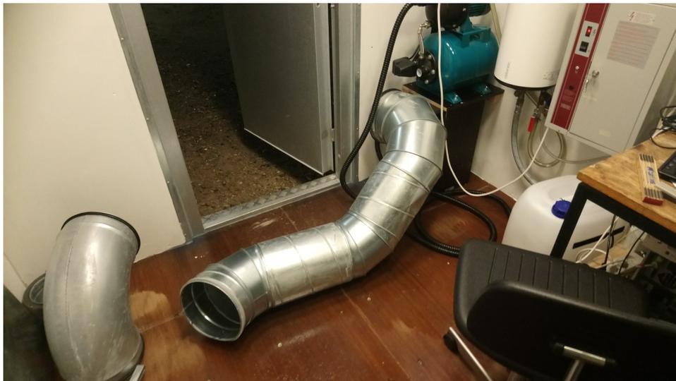
**Figure 11.7:** Duct fallen down
