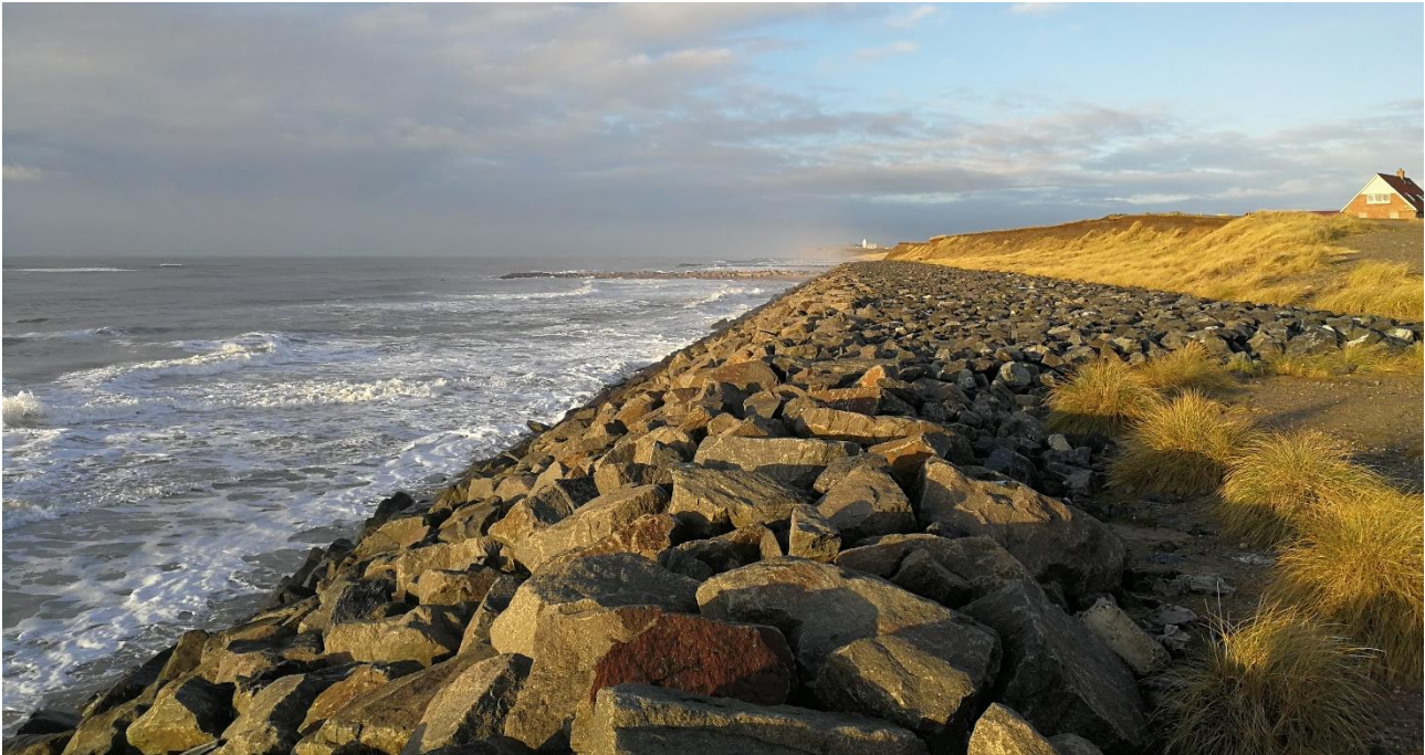
Figure 1.6 – The revetment in the picture is placed between the angled groin known as Q and the perpendicular groin known as P on the westcoast of Denmark near Fjaltring. Private photo.
