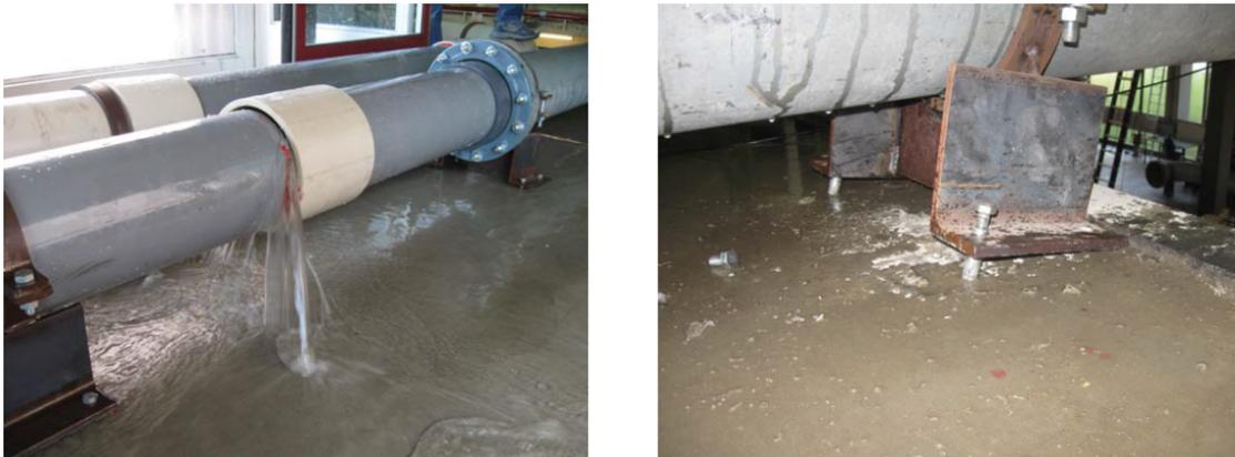
Figure 3.4: Water hammer damages at Deltares, the Netherlands. [7]
