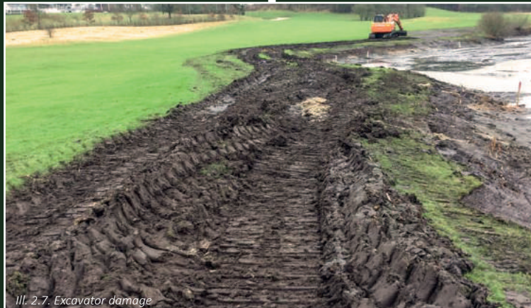
III. 2.7. Excavator damage
