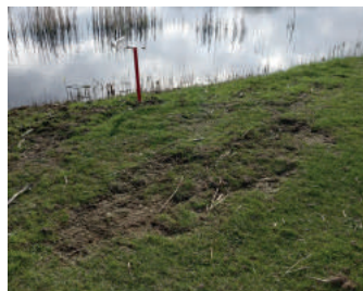
Ill. 2.57. Damage from excavator
