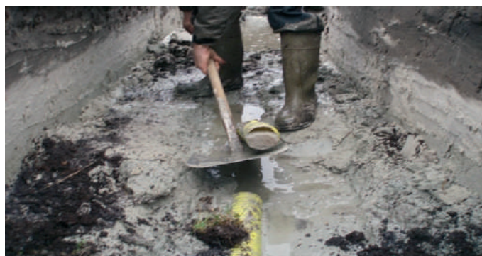
Illustration 30.5 - Sand blockage in drain.
