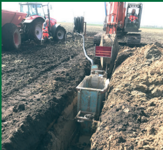
Illustration 29.3 - Drainage with excavator.
