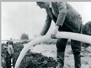
Illustration 18.3 - Plowing and PVC pipe introduction.
