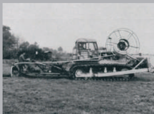
Illustration 18.3 - Plowing and PVC pipe introduction.
