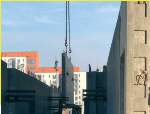
Illustration 11.1 - Lifting the concrete element.
