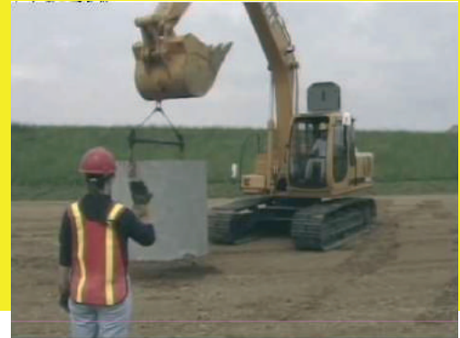
Illustration 10.3 - Communicating by hand signals to machine operator.
