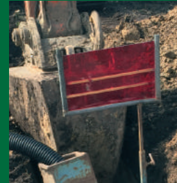
Illustration 29.2 - Leveling plate.
