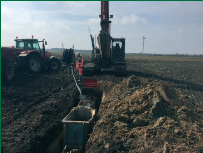
Illustration 28.2 - Placement of drain box.
