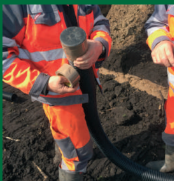
Illustration 29.4 - Tapped connection.
