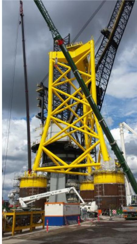
*Figure 2.6.* Installation of suction bucket jackets at the Borkum Riffgrund 1 project area [4C-offshore, 2016].
