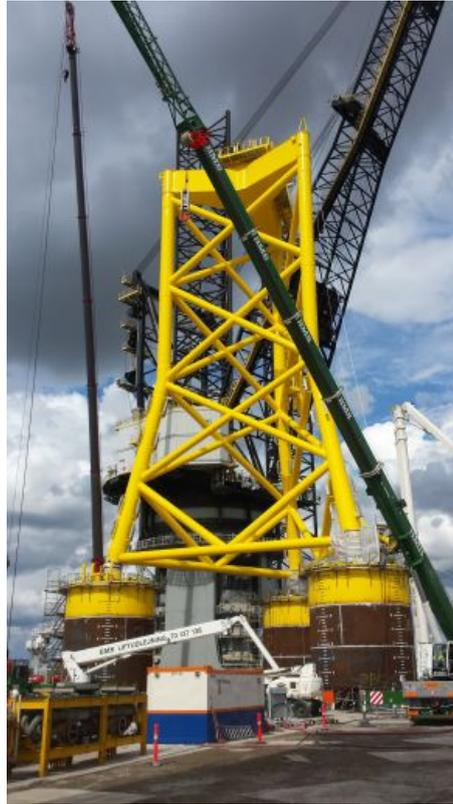
*Figure 2.6.* Installation of suction bucket jackets at the Borkum Riffgrund 1 project area [4C-offshore, 2016].
