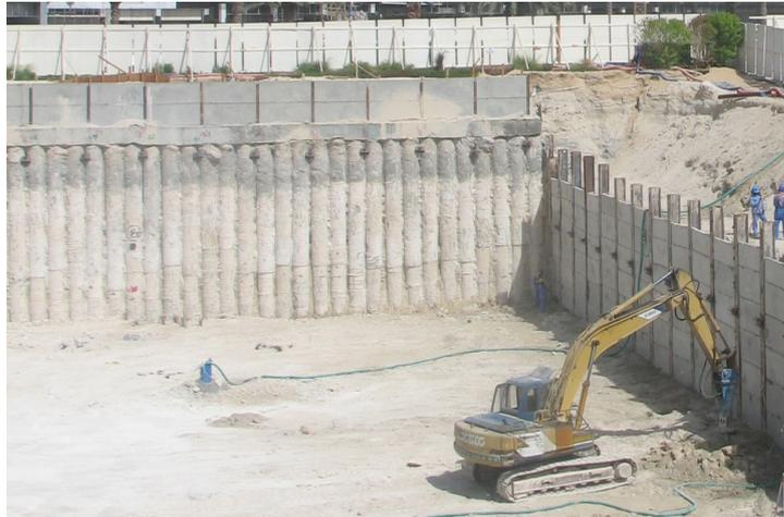
**Figure A.2:** Typical secant pile wall with one anchor level besides a soldier pile wall.[30]
