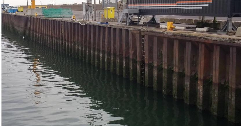
**Figure 1.2:** A quay constructed as a retaining wall in the harbour of Esbjerg.[2]
