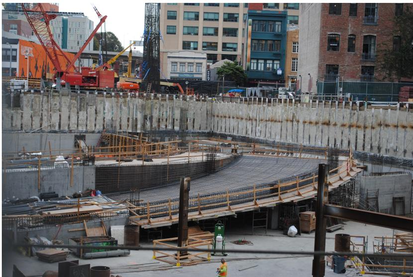
**Figure 1.1:** In land construction pit ensuring stability in a dens urban area.[1]
