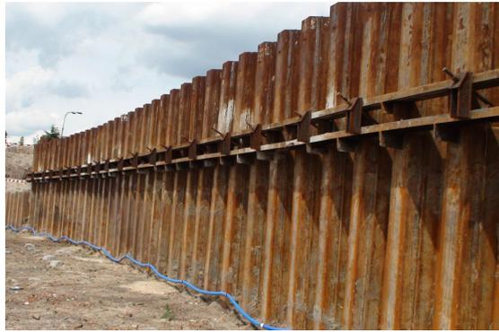
**Figure 1.5:** Typical installed sheet pile wall with an outside waling level.[3]
