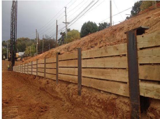
**Figure A.4:** Typical soldier pile wall.[31]
