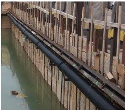
(a) Outer waling level attached on a soldier pile wall in a construction pit in Copenhagen.
