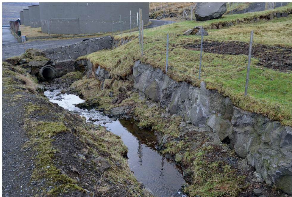
Ill.31 The stream at Niðan Horn, and how the pipe leads the water under the road and the low waterlevel there have space more
