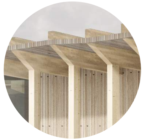
Roof beam meeting the columns of the courtyard
