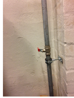
(b) Valve controlling the water tank.
