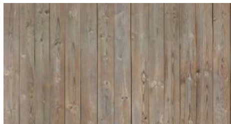
Illustration 2.15: Spruce used as interior wood cladding in the main building
