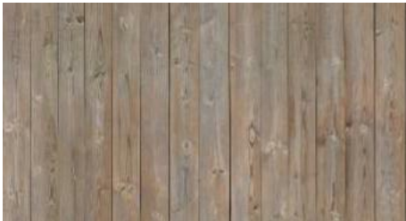
Illustration 2.5: Spruce used on the facades. Before commissioning it is dry treated so the pore will close which will create a longer lifetime
