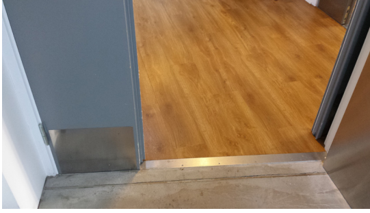
III. 5. Doorstep inside the building
