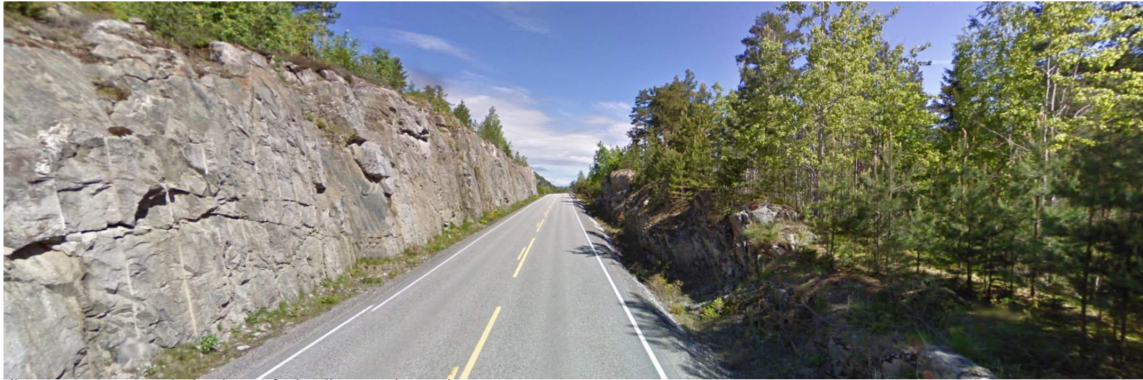
Ill. 16 Deep cuts in the landscape for levelling out the road
