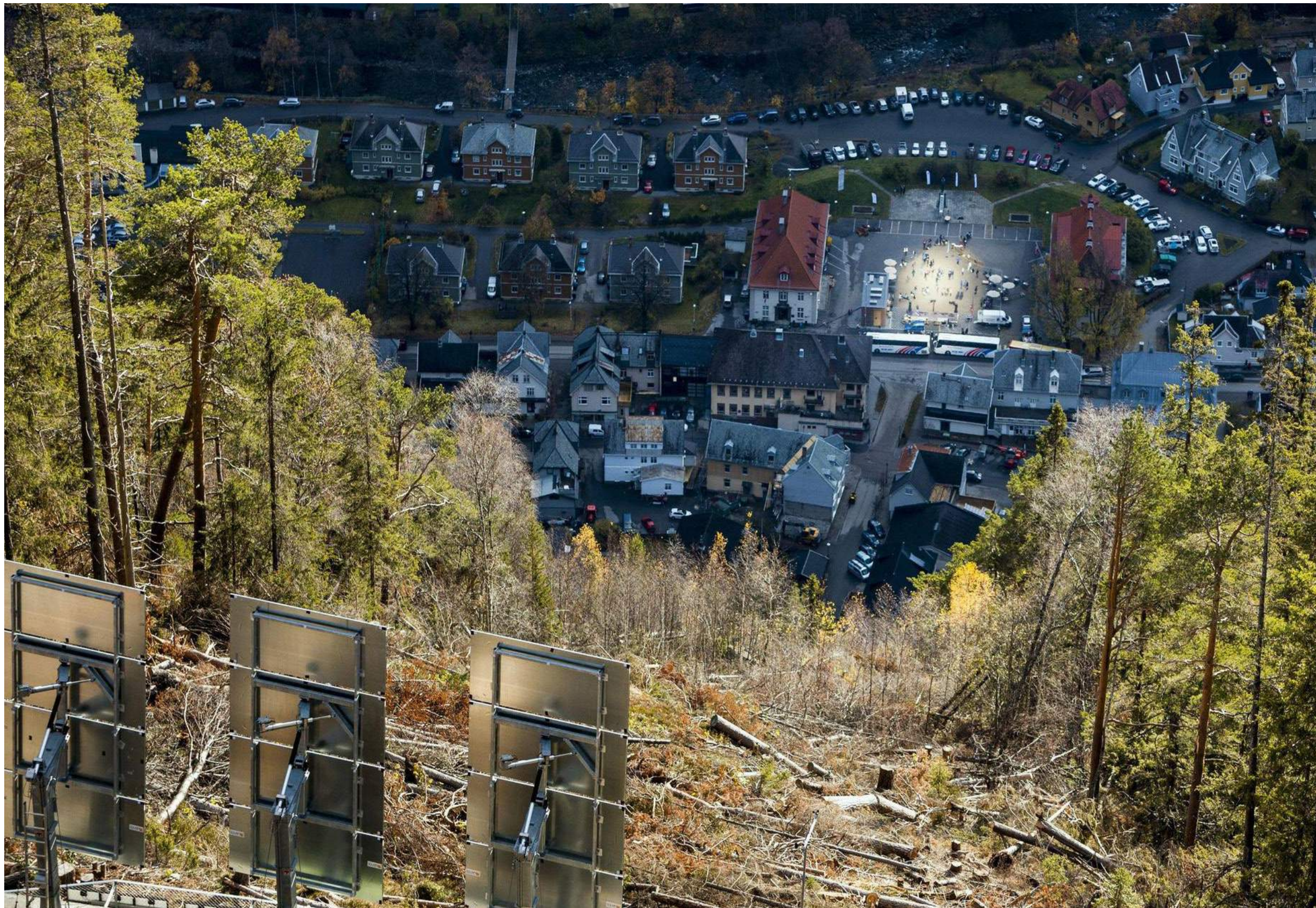
III. 10 Mirrors reflecting daylight onto Rjukan Town Square
