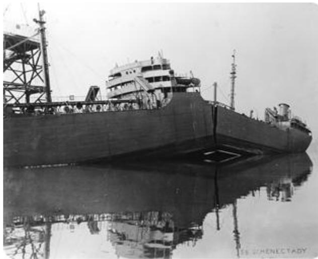
*Figure 1: Liberty ship exposed for fracture*
