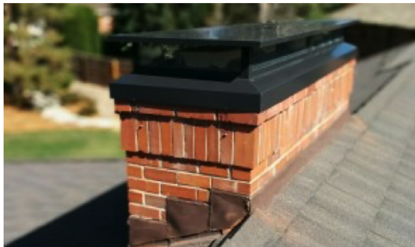
Figure 4.39. Venturi ventilator. [Master Services]
