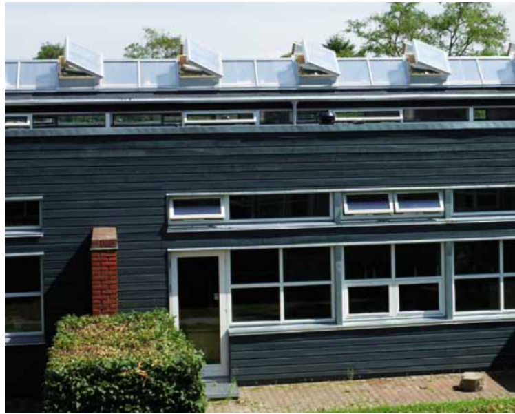
Figure 4.34. The hinged windows for the outer rooms are placed above the large window sections in the facade. The openings for the inner rooms are the roof windows together with the series of openings just below. [WindowMaster, b]
