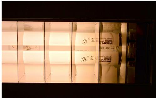
*Figure H.2.* The two 35W fluorescent light tubes in the armature
