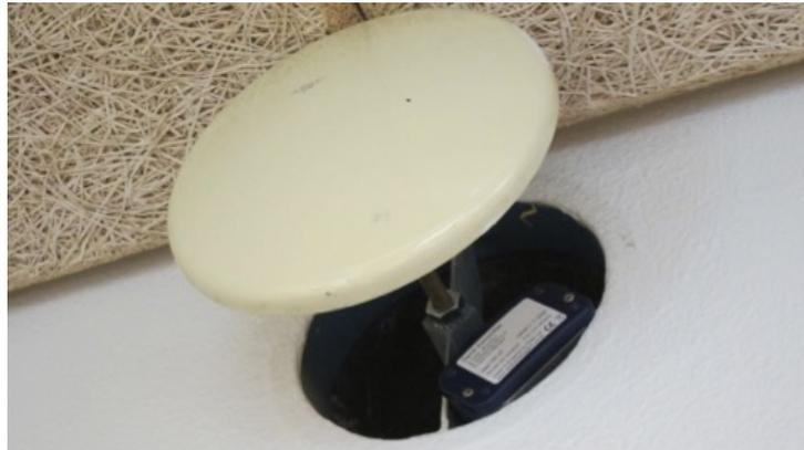
Figure 2.11: Eltek GD47 wireless transmitter located in exhaust opening measuring air temperature and CO<sub>2</sub>-concentration.
