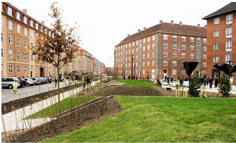
Figure 3: Example of climate adaptation (Sustainable Urban Drainage System) SUDS solution in Tåsinge Plads, Østerbro, Copenhagen.
