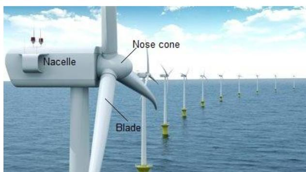
**Figure 16: Offshore Wind Turbine Parts (Shutterstock, n.d.)**
