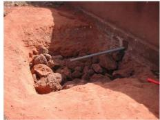
Figure 49: Open soak pit with installed PVC pipe (Sswm.info, 2015)
