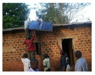
Figure 64: Solar PV being installed on a house : (Sunlabob. com, 2015)
