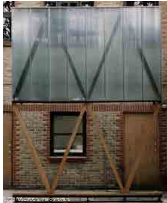
Ill. 70 - Polycarbonate and structure
