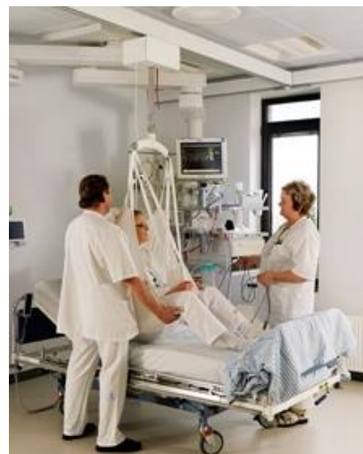
Figure 2-2 Hoist System in use at hospital
