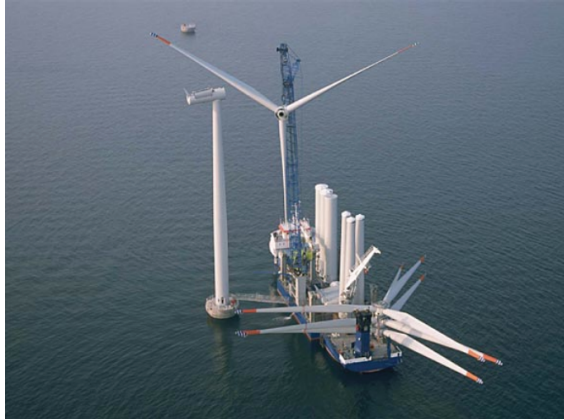
Figure 2.2. Installation process with onshore pre-assembled components. [Guillen et al., 2011]
