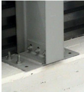
**Figure 4.5.** Plate attached to the end of the column.[Constructalia, 2014]
