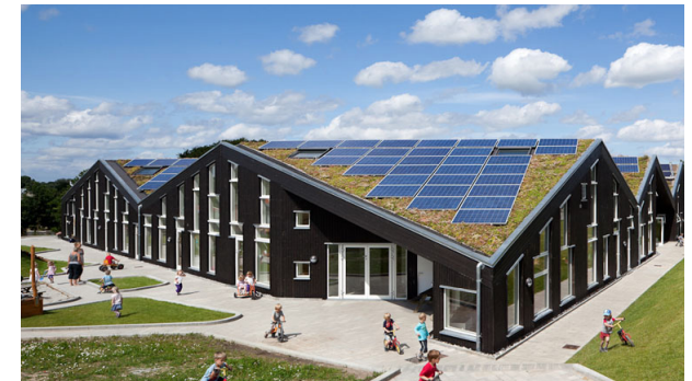
ILL. 03.20 THE ROOF STRUCTURE COVERED WITH SOLAR PANELS
