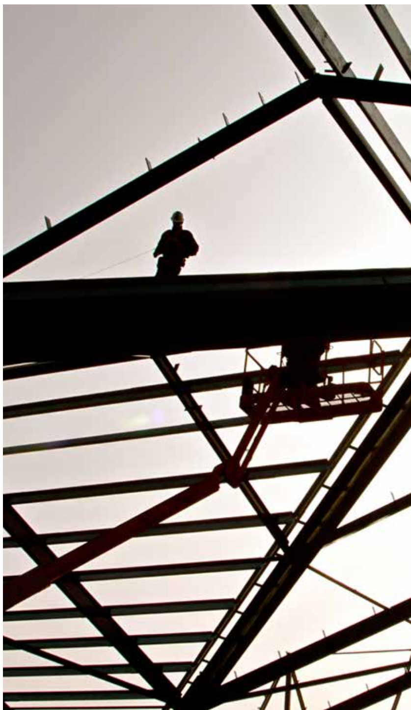
Fig. 10. Building the structure at Vejlskovgård
