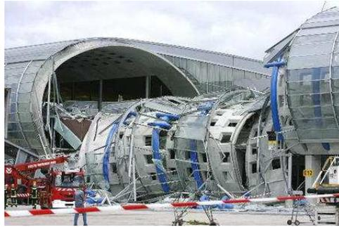
**Figure 1.7:** Partial collapse of the Charles de Gaulle Airport Terminal, Paris.
