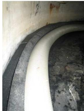
(b) Joint between tank wall and membrane.
