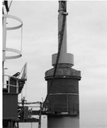
Pile in drive gate with hammer in place
