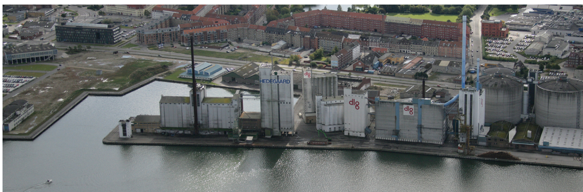
ill. 01 Østre Havn as seen from north
