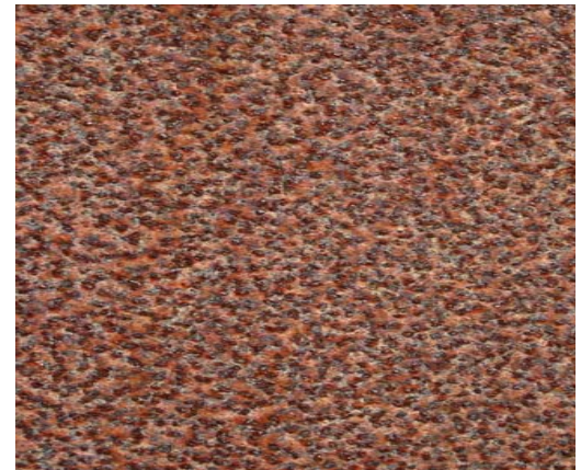
Fig.86. Rust coated metal
