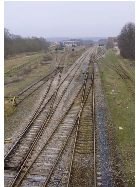
Fig. 26. The Railway track creates a barrier
