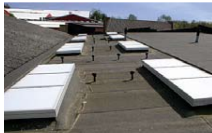
ill. 1.131 - Plane PC skylight with fire ventilation from Primalux. On the right an open module from a light row is shown.
