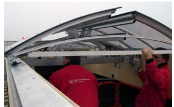
[ 18 ] The opening function is checked. Potential alignment inaccuracies in the mounting is corrected and all bolts/screws between the frame, motor and opening modules are securely fastened.
