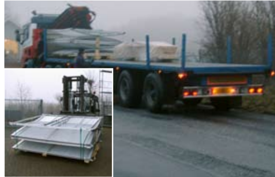
[ 2 ] The materials for the lightrow arrive by truck and are unloaded with a forklift.
