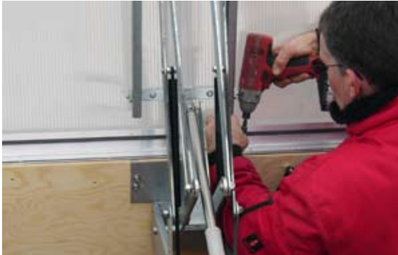
[ 19 ] The opening module is opened completely. Following this the alu profiles of the opening modules that rests on the side frames can be fastened to the side frame.
