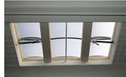
ill. 1.27 - Vaulted PC fire ventilation skylight from Optilite. Note the different measurements of the two types of windows in the cluster and the fact that the middle window has no motor.
