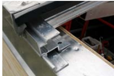
Outside alu profiles touches inside alu profiles with no change in material which produces a thermal bridge.
