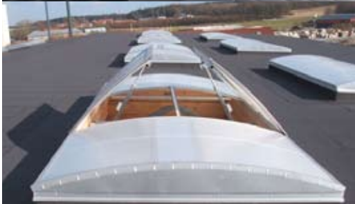
PC skylight with fire ventilation on flat felt roof
