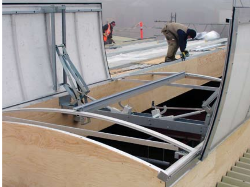
ill. 2.12. - The current motor is placed across the window, which decreases the inflow of light into the building. Furthermore this solution increases the perceived aesthetic complexity.
