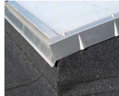
A detail shot of the corner.
