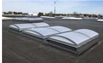
ill. 1.27 - Vaulted PC fire ventilation skylight from Optilite. Note the different measurements of the two types of windows in the cluster and the fact that the middle window has no motor.
