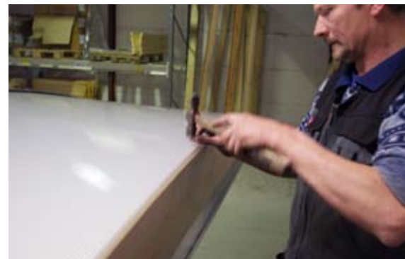
[ 24 ] The fixed PC plates are nailed to the wooden endgables.
