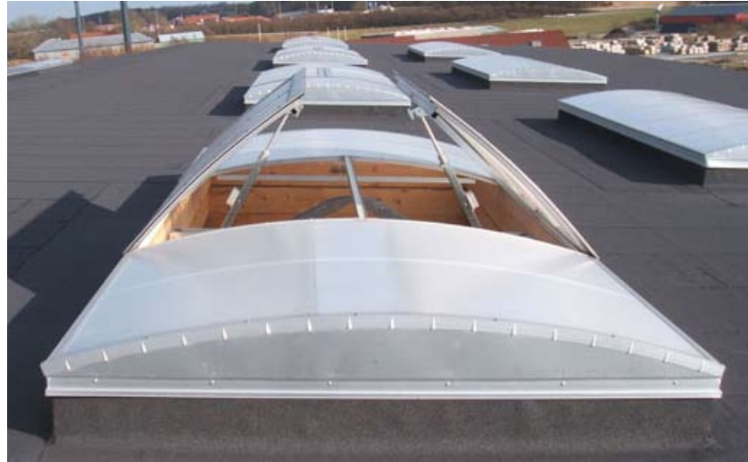
Vaulted PC skylight with fire ventilation - during opening sequence
