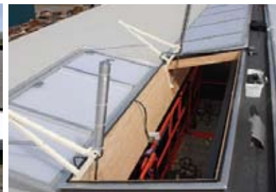
ill. 1.131 - Plane PC skylight with fire ventilation from Primalux. On the right an open module from a light row is shown.
