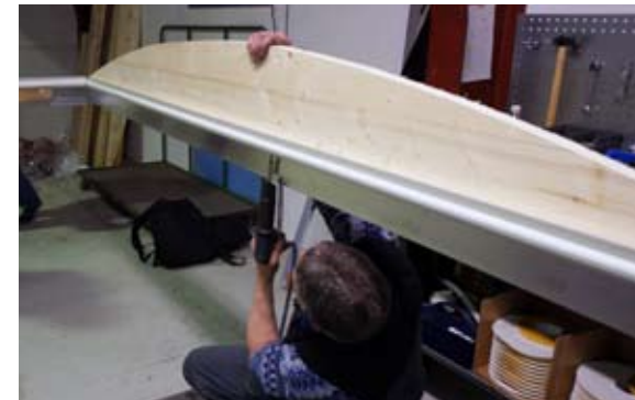
[ 12 ] A wooden end gable is mounted onto each short end of the alu frame.
