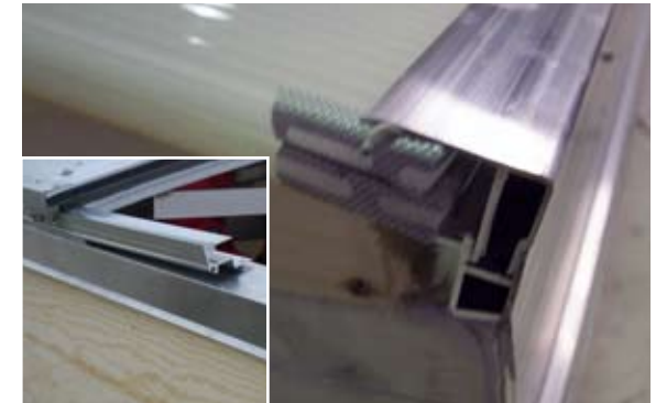
[ 24 ] Subsequently the fixed PC plates are mounted onto the distance alu profiles in the same way as in the assembly of the pre-assembled window. (Large picture taken from the pre-assembled window).
