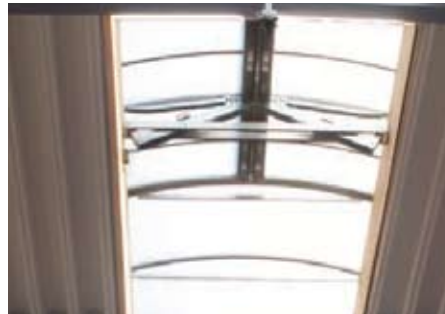
ill. 2.12. - The current motor is placed across the window, which decreases the inflow of light into the building. Furthermore this solution increases the perceived aesthetic complexity.
