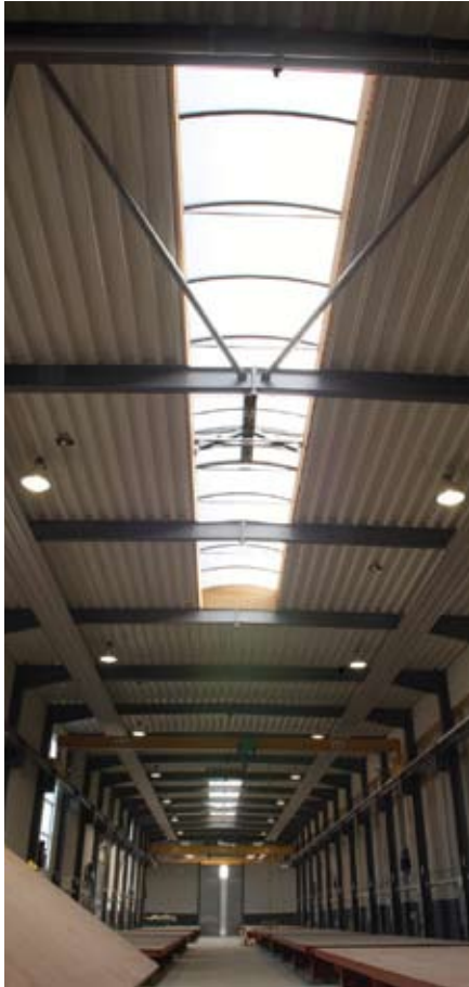
The vaulted PC lightrow with fire ventilation seen from inside.
