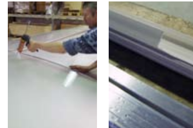
Cutting away material and applying extra material when assembling the skylight.
