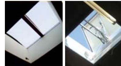
ill. 1.38 - The two types of skylights shows from inside.
