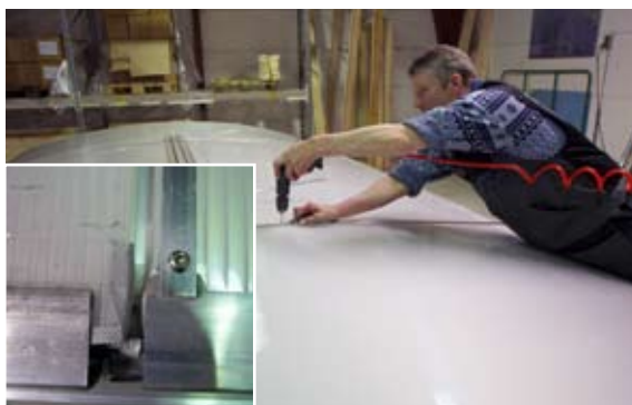
[ 17 ] In the meeting between the opening PC plates and the fixed PC plates, an alu profile is mounted on top of the opening PC plates. This is done to secure these PC plates to the frame of the opening module.
