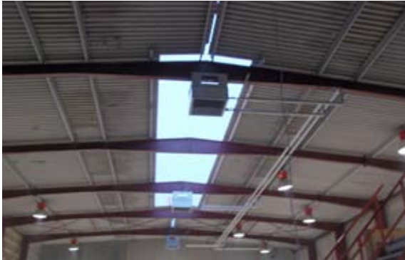
[ 1 ] The hole for the lightrow has been cut prior to the delivery of the assembly kit from Domex.
