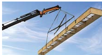
ill. 1.132 - A light row lifted into place.
