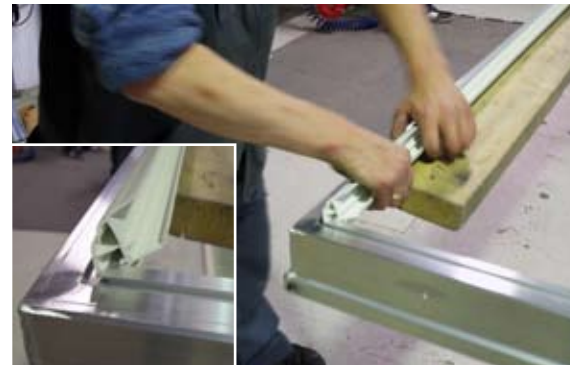
[ 3 ] Plastic profiles for collecting condensation and reducing thermal bridges are clicked on in one end of each long side.
