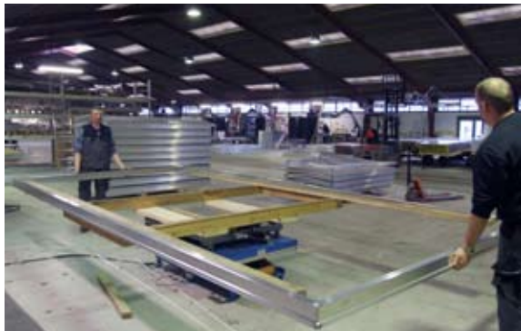
[ 1 ] A welded alu-frame is placed on a workbench.
