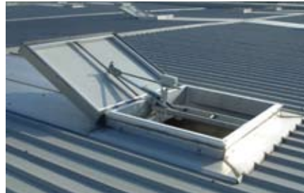
ill. 1.36 - The two types of pre-assembled skylights - A hinged model and a sliding model. The two types comes in Flat, Ridge and Vaulted.
