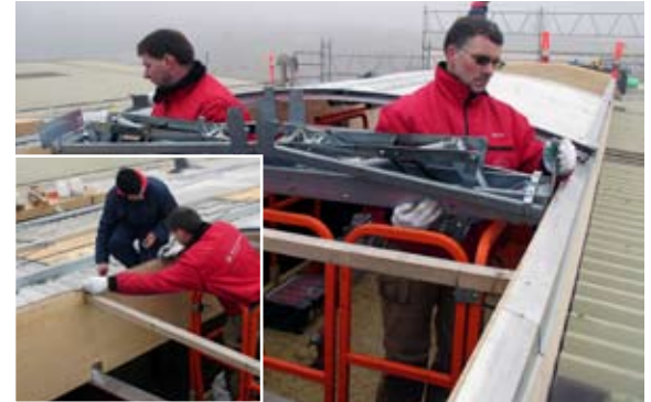
[ 12 ] The position of the motor is measured and the motor is loosely placed - resting on the side frames and secured with one or two screws.
