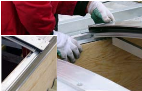
[ 22 ] When positioning this opening module like in [ 13 ], the opening module is slid into the alu profile mounted in [ 20 ].
