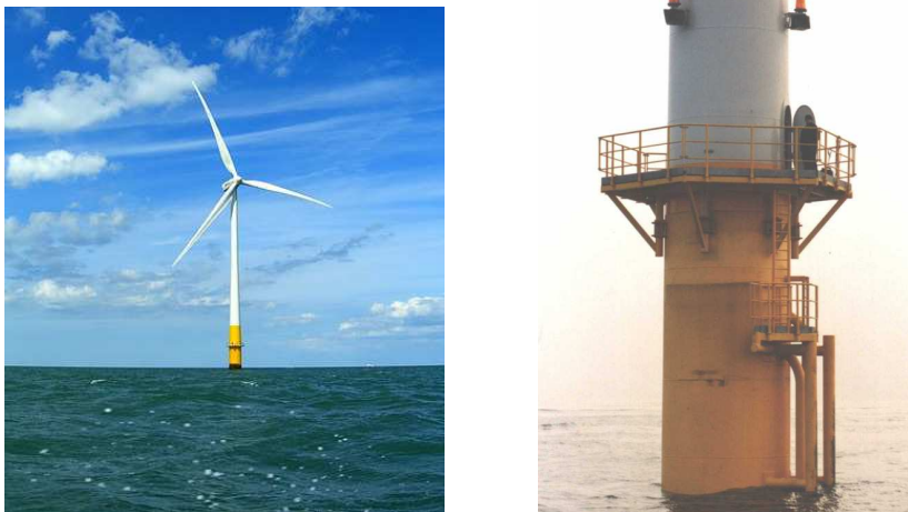
Figure C.1. To the left is an offshore wind turbine from Farm1 (2007) and to the right a close-up of the landing stage and the platform running around the exterior of the turbine substructure from Oceanatlas (2007).
