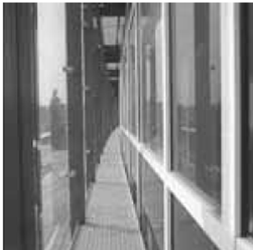
Figure 1.1 Example of double skin façade construction. [2]
